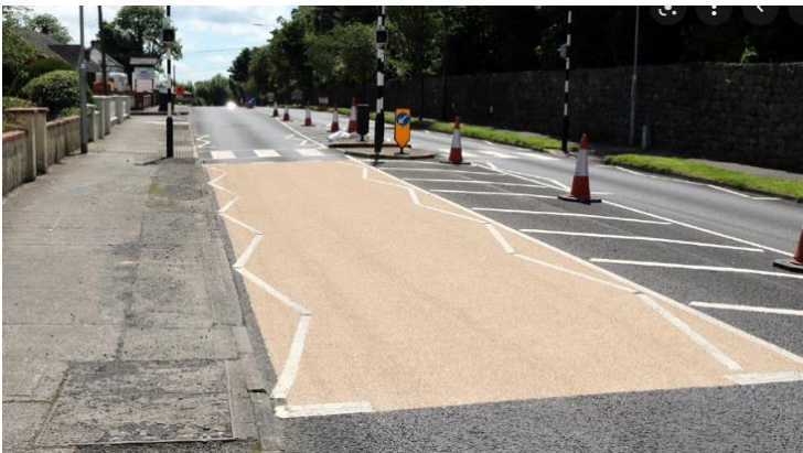
Pedestrian crossings and anti-skid surfacing
